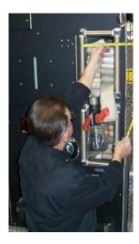
**Step A =** Measure the **width** of the speedlay opening from the *inside of the compartment* as show here. Your dimension =
